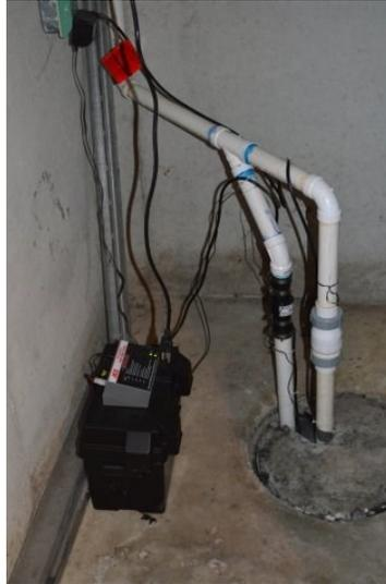
Sump pumps are self-activating electrical pumps that protect homes from water intrusion. They are usually installed below basement or crawlspace floors in a sump pit to remove rising groundwater and surface runoff before it has a chance to get into the home. Pedestal pumps which sit above the water line and are not designed to get wet, submersible pumps that sit at the bottom of a sump pit and are designed to be underwater.
